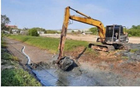
River dredging work (SGS)
